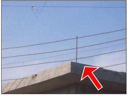
Constructing house very near to electrical lines – Not leaving the mandatory clearance of 1.2 meters in case of LT network as per rule 80 0f Indian Electricity Rules 1956.
